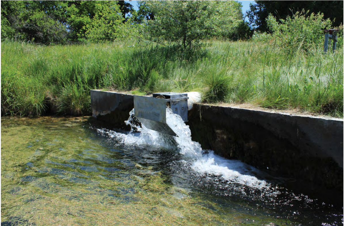
Figure 6. Inlet structure during normal operation (splashplate in down position).
