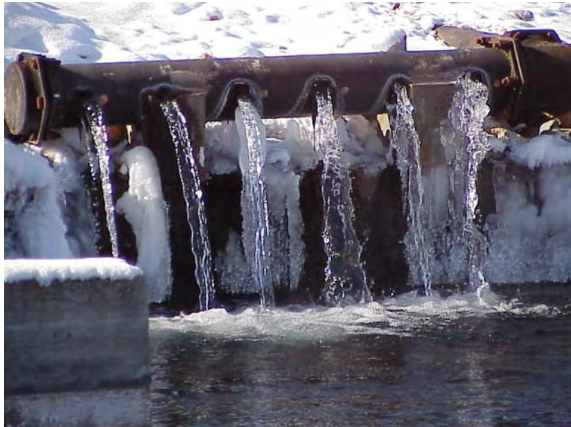
Figure 2. Cast iron pond inlet used as a pond inlet at McNenny State Fish Hatchery. This image shows only one-half of the symmetrical structure.
