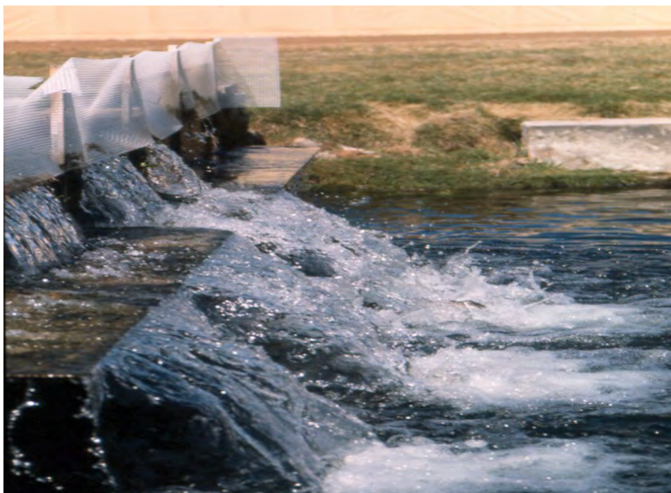
Figure 1. Wooden headbox with a metal splashplate initially used as a pond inlet at McNenny State Fish Hatchery (note the plastic mesh attached to the headbox to try and prevent fish from ascending into the inflow pipe, as well as the fish jumping up the turbulent water towards the headbox).
