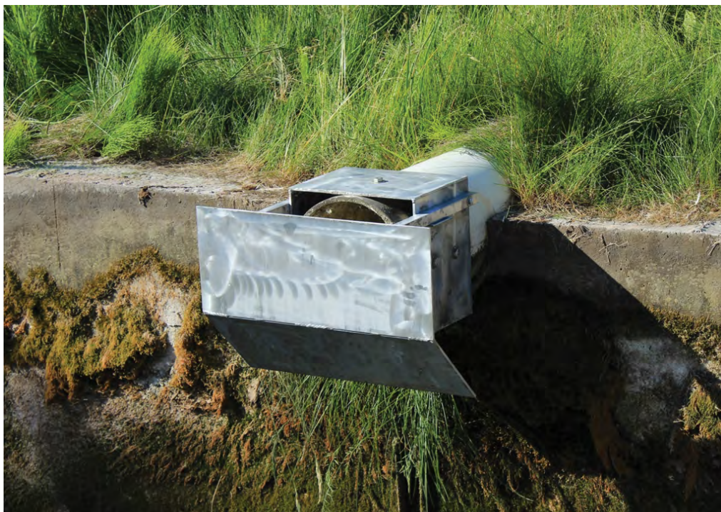
Figure 3. Novel inlet structure with splashplate in the down position.
