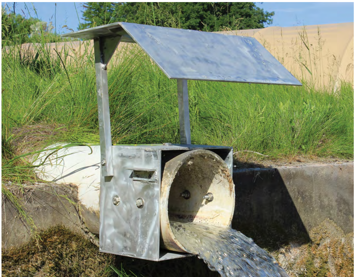
Figure 7. Inlet structure during cleaning, with splashplate in the up position.
